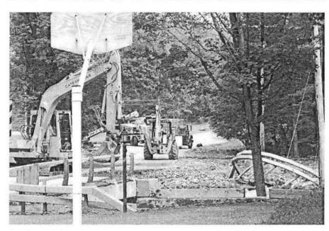
By June 30th, road crews with machinery were already at work repairing the flood damage to the County Route 10 bridge over Kortright Creek. The bridge itself is intact, but the flood washed away part of the road in front of the bridge. Note the bent guard rail on the right.
